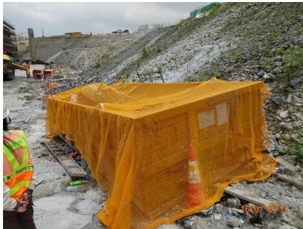
Exposed surface was covered by cement mortar
