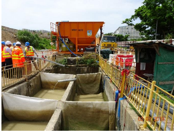
Q6: Wastewater treatment facility 24 cu. m.
