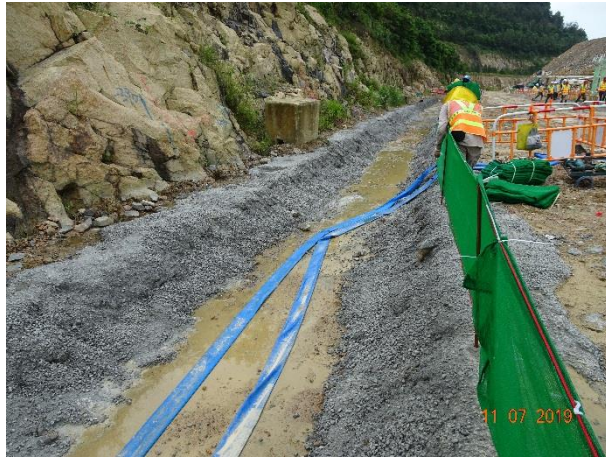
Perimeter channel to collect site surface
